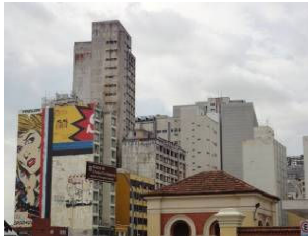
Picture 13: Deteriorated buildings subject to reconstruction
