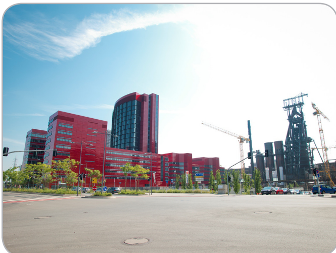
Belval - former steel works and new constructions
