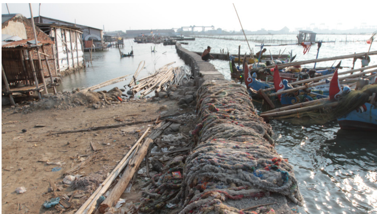
Picture 4. Flood retaining embankments built by local government to withstand flooding. However, the tidal flood keeps affecting community's settlement. Semarang, Indonesia, Tambor Lorok community © Kota Kita
