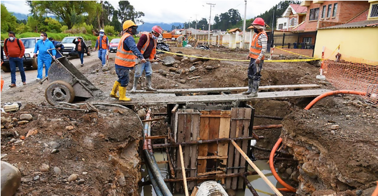
Picture 15. Cuenca. PB Works in villages © Cuenca Municipality
