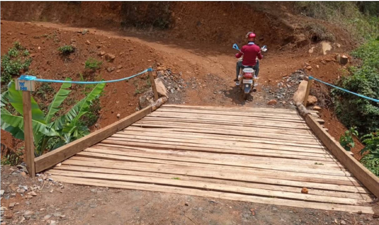
Picture 16 & 17. Luhwindja, South Kivu Region, bridges. Before and After PB. © Espérance Mwamikazi Baharanyi
