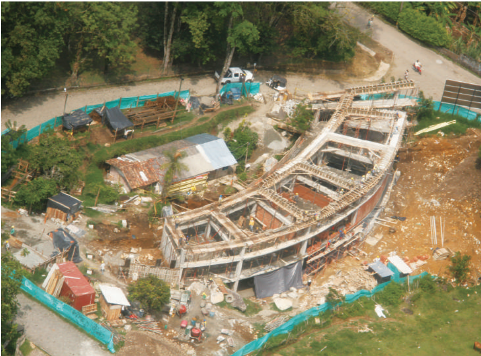
□ Construction of an Educational Thematic Park in the Antioquia
