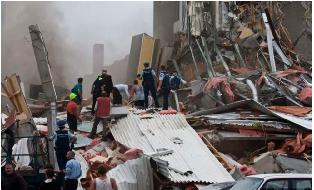
□ Post-earthquake Site of Christchurch
