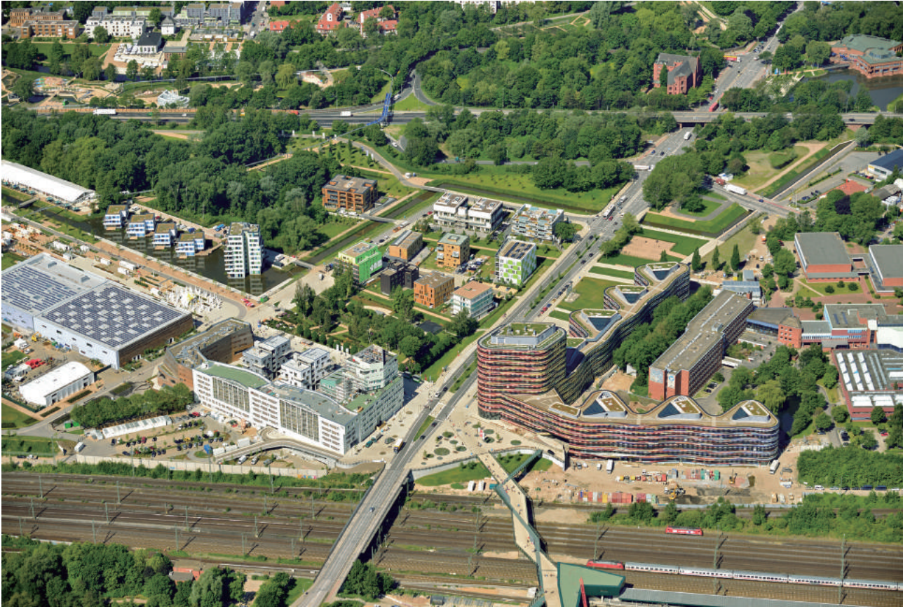
□ Energy and Network Center in Wilhelmsburg, Hamburg
