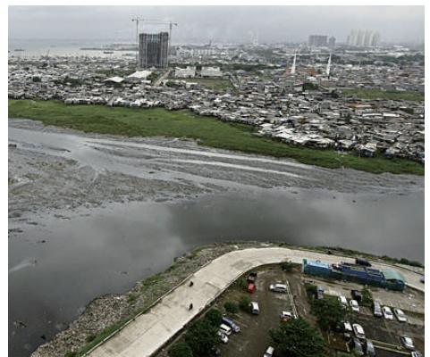
□ A large number of sediments in Pluit Reservoir
