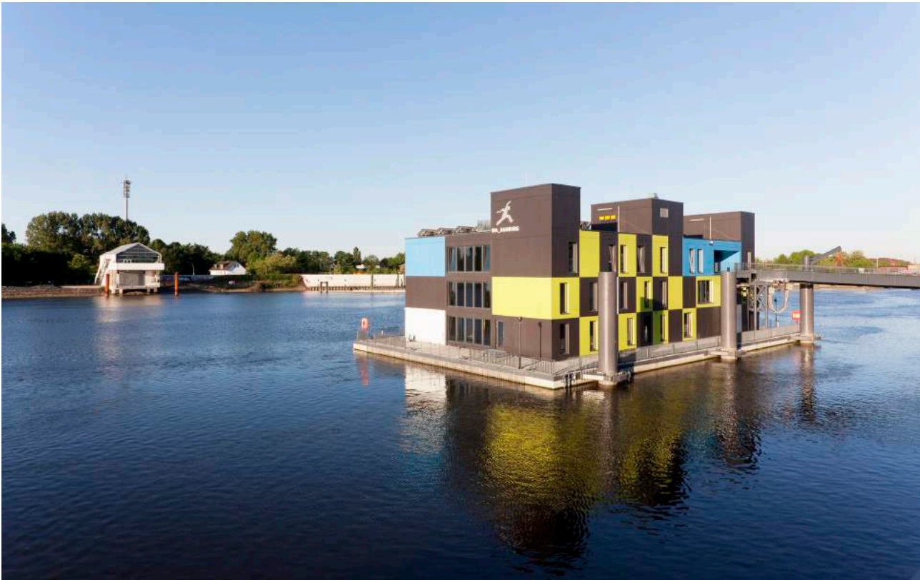
□ The International Building Exhibition (IBA) Hamburg brings out three-layer Dock building, floating up and down as the Elbe's tide rises and ebbs.
