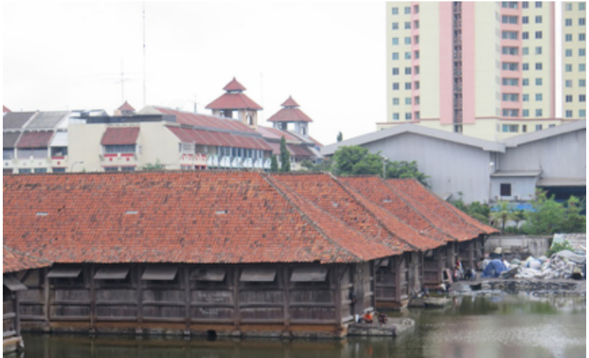
The 19th century wooden floating warehouses
