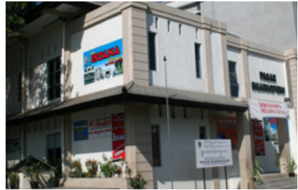
Image before and after the refurbishment of the Ngasropuro Electronic Market Source: City of Surakarta
